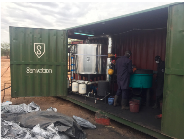
FIGURE 5: TREATMENT AND BRIQUETTE FACILITY DESIGNED IN A SHIPPING CONTAINER
