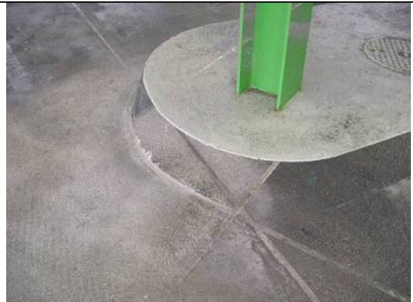
Sealed joints in good conditions
