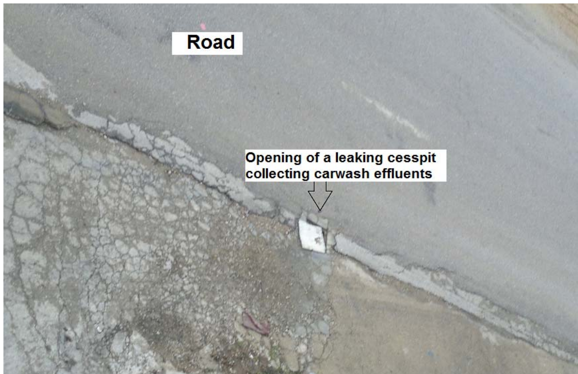
Photo 7: Opening of the cesspit collecting carwash effluents, located on a road's limits.
