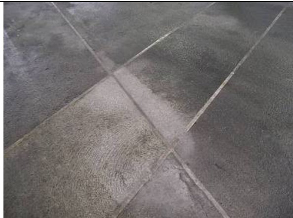
Sealed joints in good conditions
