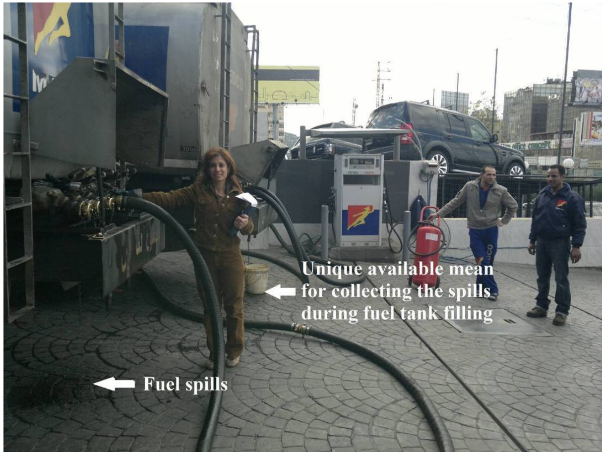
Figure 28: Spills while filling underground fuel tanks
