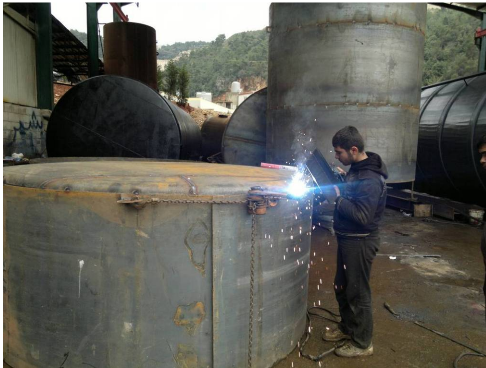
Figure 17: Joining the tank concave extremity by welding.
