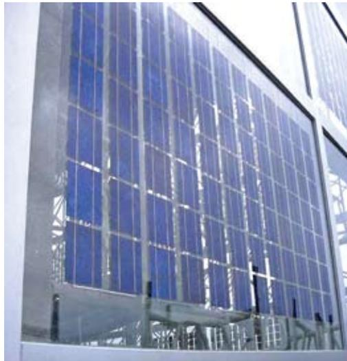
**Figure 15. BIPV modules integrated into a façade**
