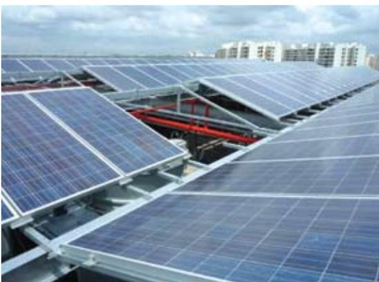
**Figure A.8.2. Partially completed PV array**
