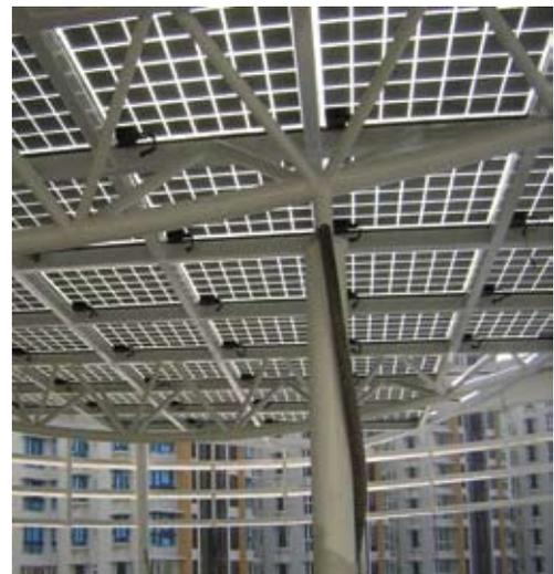
**Figure 16. BIPV modules integrated into a skylight canopy**
