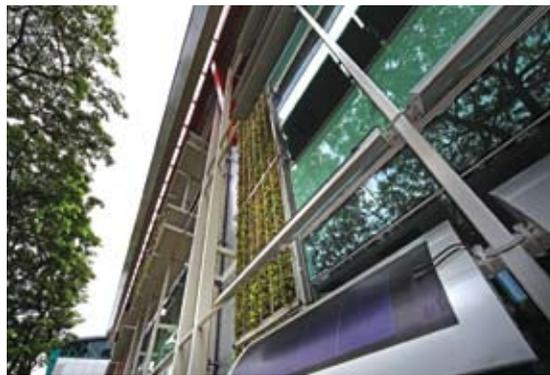
Figure A.1.2. PV array view (PV Sunshade)
