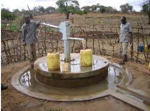
Handpump on shallow dug well
