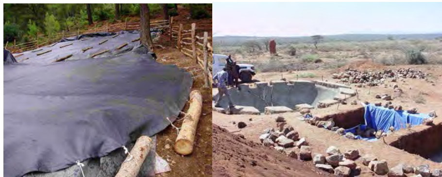
Runoff water collection
