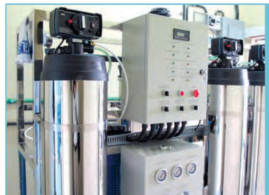
Reverse Osmosis Treatment
