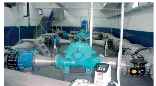
A pumping station after modernisation
