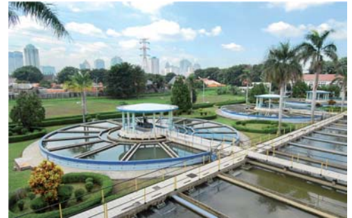
Rehabilitated Pejompongan water treatment plant
