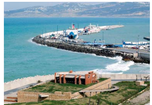
The new wastewater treatment plant
