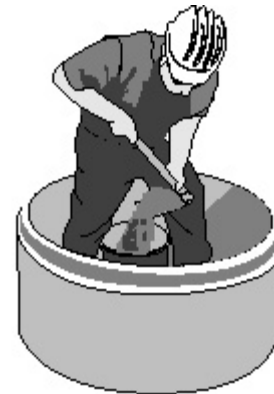
Filling Bucket with Digging Hoe
