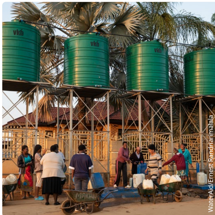
Community members fetching water at the water points underneath the recently built elevated water storage tanks in Ha-Mangilasi, Vhembe district, Limpopo province, South Africa.
