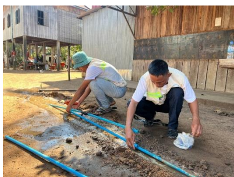
Fig 16. The AEPSS technician with the WMC of Sala Visai is repairing a leak on the pipe.
