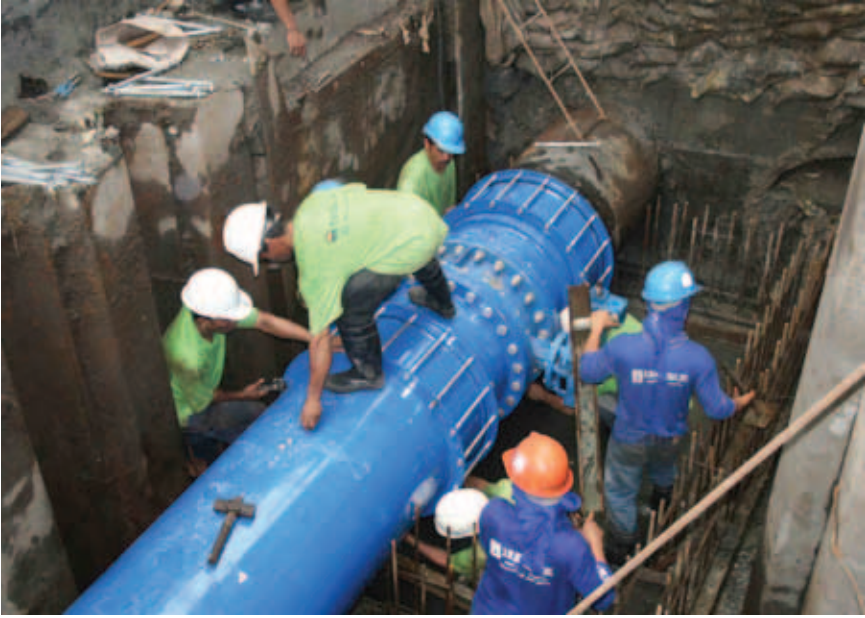
Maynilad contractors at work during an interconnection activity in Sta. Mesa, Manila. Photograph courtesy of Federico Juane, Maynilad Water Services.
