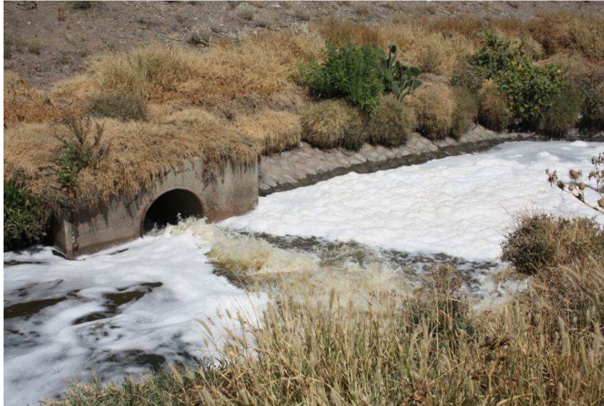
WWTP Outflow/ Bypass, Sanaa, Yemen - Part of the wastewater is not treated and flows through a bypass where it is mixed with the treated effluent.
