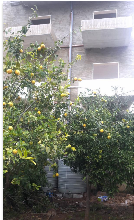
Figure 1. Rainwater harvesting system installed by ACTED on a residential building in Bergayel, Akkar.
