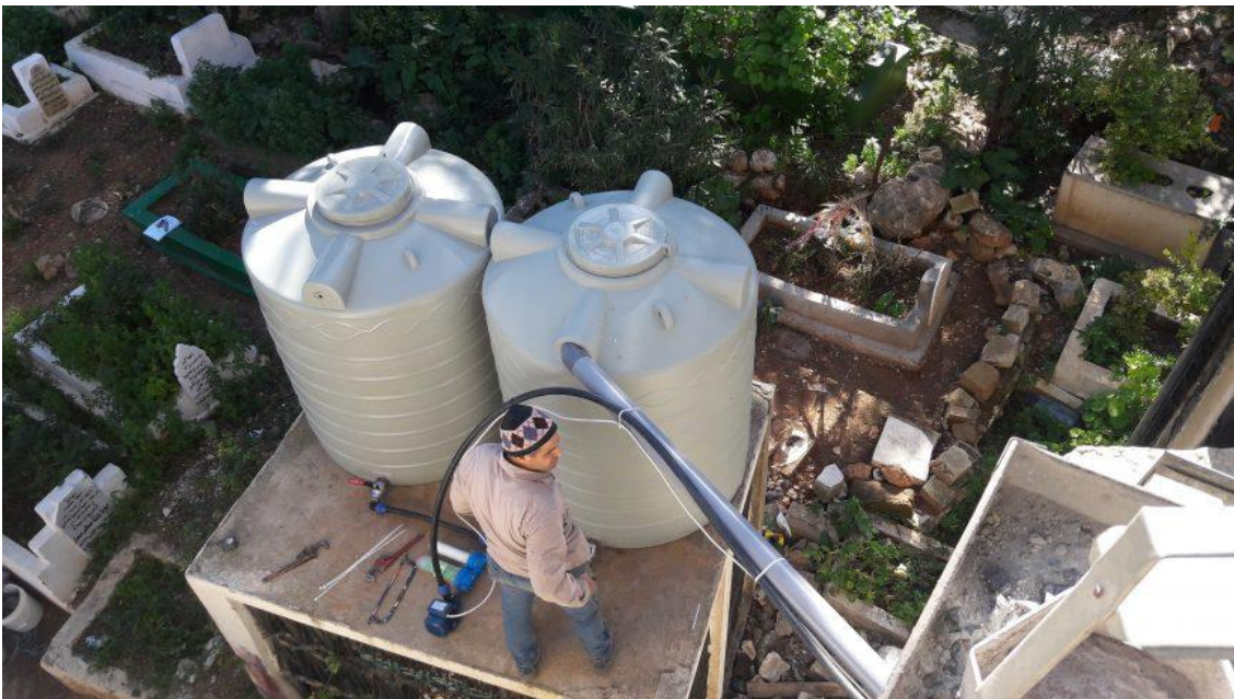
Figure 3. ACTED installation of rainwater harvesting system in Berqayel, Akkar
