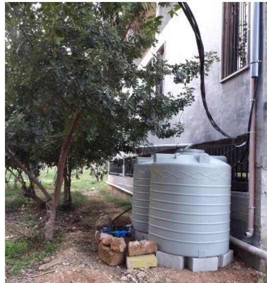
Figure 4: Rainwater harvesting systems installed in the municipality of Berqayel, Akkar.
