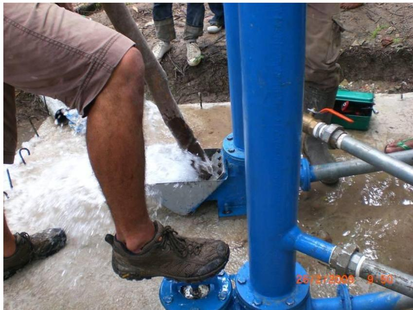
Figure 26: Priming the Hydraulic Ram Pump
