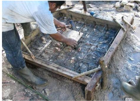
Figure 7: Construction of pump basement, NTT
