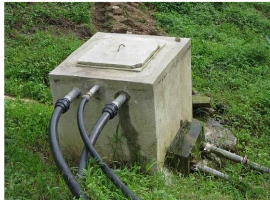
Figure 5.b: Header tank for 2 pumps from AID Foundation
