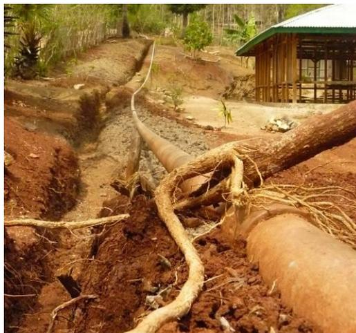
Figure 21: Burring delivery pipe
