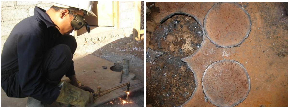
Figure 28: Cutting the iron plate
