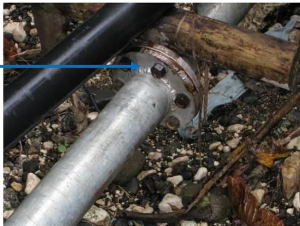
Figure 6: Drive pipe and flanges
