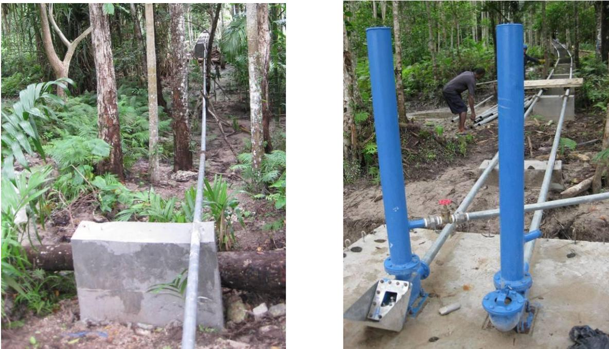
Figure 23: Drive pipes and supports
