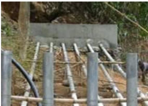
Figure 5.a: Header tank for 6 pumps from AID Foundation
