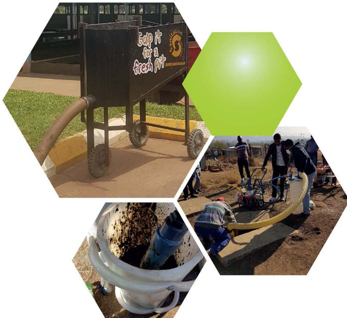
▲ Figure 4 : **Semi-mechanized pit emptying**
