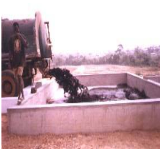
Plate 4-1 Septic Emptyer Discharging into the Sludge Storage Chamber
