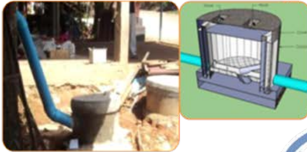
1. Connection box: DN 60 mm
