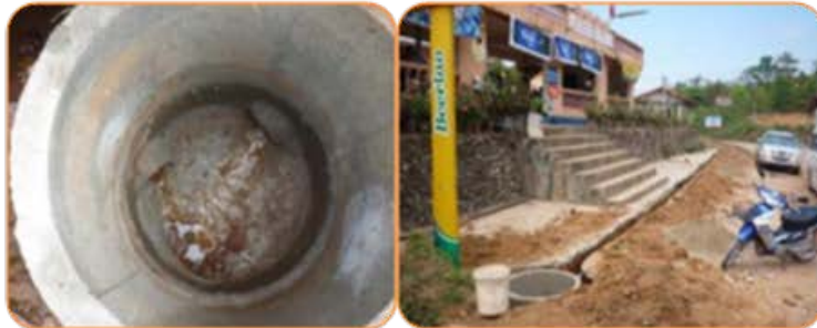
2.1- Sewer: uPVC DN100 mm: 1,043m - 46 manholes DN80 mm
