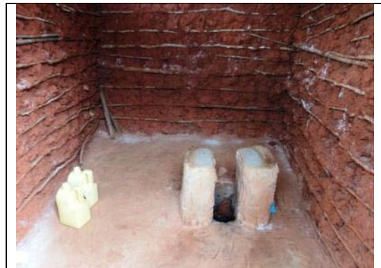
Figure 23 Toilet with raised sitting blocks (Chege 2012)
