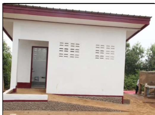
Figure 31: Prototype primary school latrine and water supply, Phongsaly province. (Badloe, 2012)
