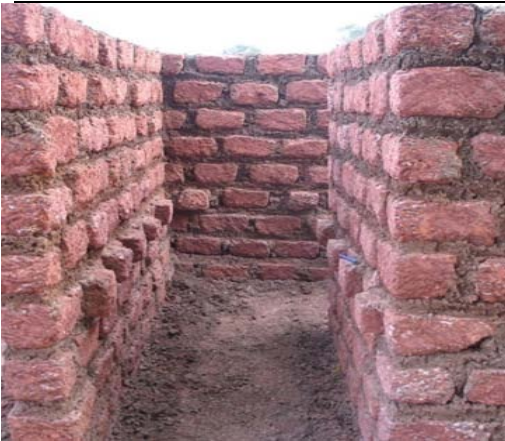
Figure 18: Protruding bricks for support to enter/exit a latrine (Kamban and Norman 2013)
