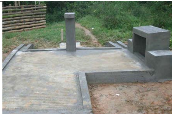
Figure 14: Water point apron under construction. Note laundry area and ramp access. (BESIK ndb)
