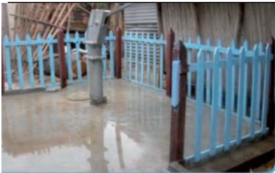
Figure 10. Example of accessible water point showing wide circulation area (WaterAid Madagascar 2010b).
