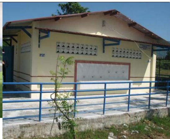
Figure 35: Latrine in Phuoc Tan Primary school, Ninh Thuan province (Nguyen and Tran 2012)
