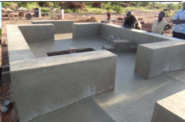
Figure 7: Accessible handpump apron, Moribila Zounoukan. Seating block is visible (World Vision Mali)
