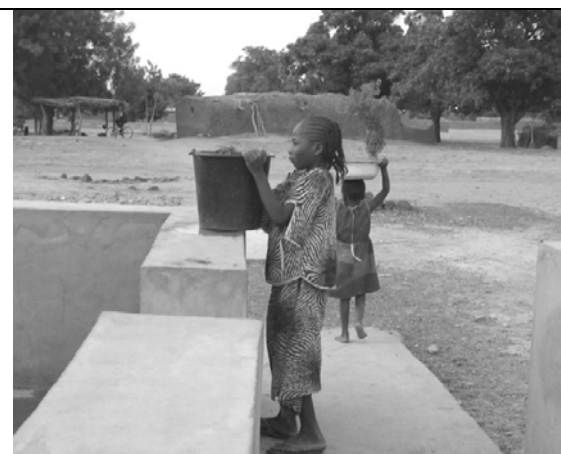
Figure 9: Low enclosure wall can be used as mid-point for resting water container. (Norman 2010)
