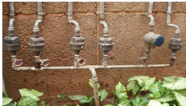
Roof tanks with faulty float valves and aging meters are two sources of meter under-registration.
