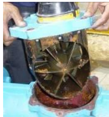
Sedimentation is a major cause of meter reading inaccuracies.
