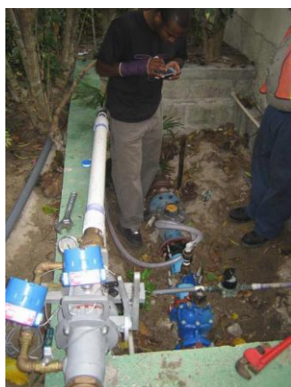
Checking accuracy of a large customer meter.
