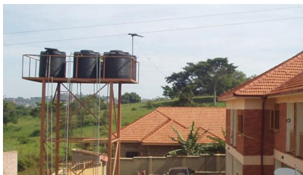
Roof tanks with faulty float valves and aging meters are two sources of meter under-registration.
