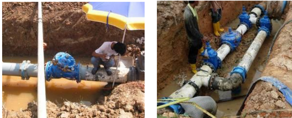
PRVs installed in meter chambers.
