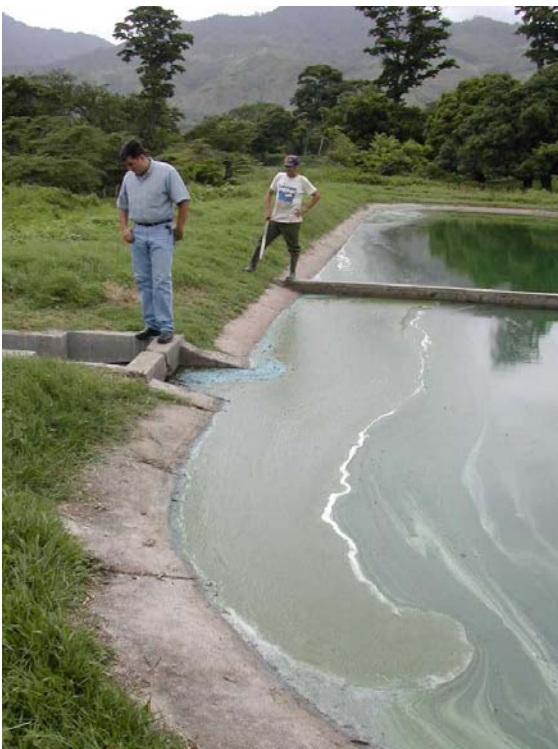
Maturation pond Scum and grease accumulation near the outlet
