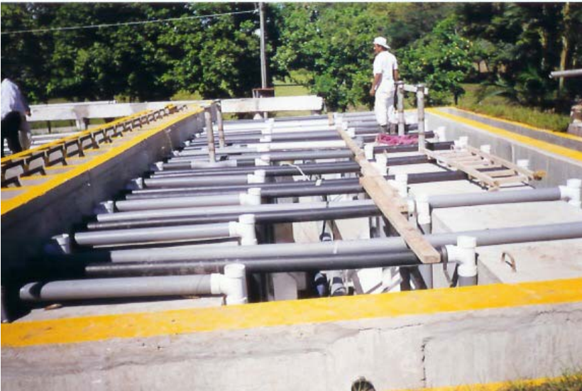
Influent flow distributed at the top of the reactor (sliders + horizontal pipes and ...
