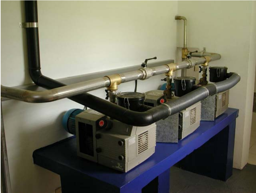
3 blower units - each 3.5 kW for 1000 PE and one unit stand-by
