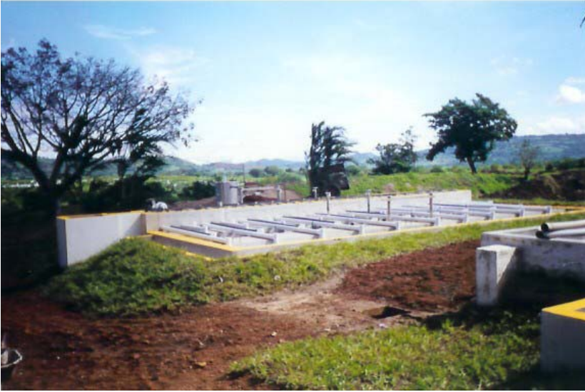
View of the compact UASB reactor.
