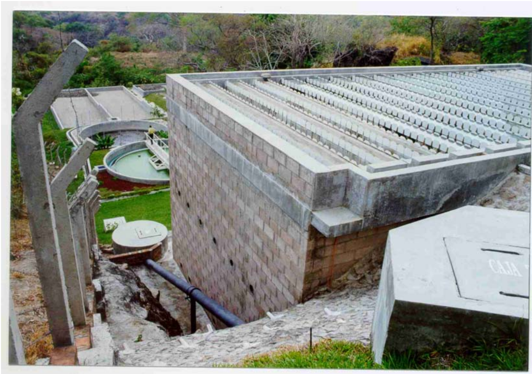
From right to left: trickling filter, sedimentation tank, sludge digester, drying beds
