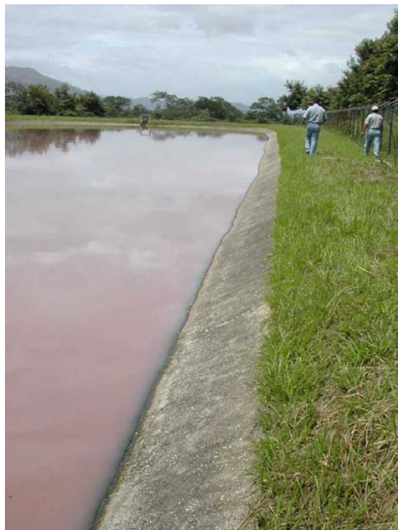
Facultative pond Anaerobic conditions prevail, consequently proliferation of rose red sulphur bacteria
