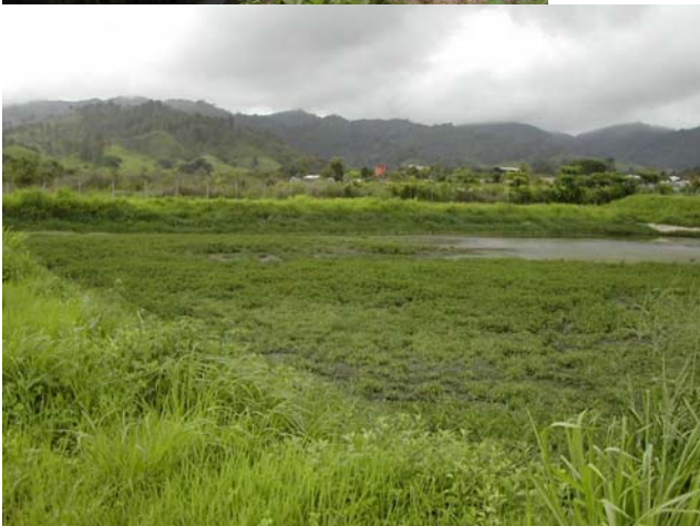
Maturation pond Poor maintenance + poor hydraulics (short circuit flow)
