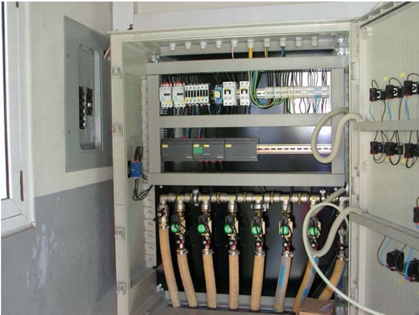
Control unit – storage programmable control in the middle and electromagnetic valves directing pressurized air to the individual consumers (fine bubbles aerators, airlift pumps for clarified water and waste sludge)
