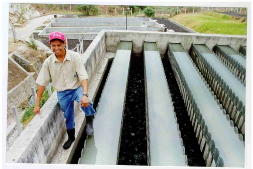
Above: on the head of the trickling filter TF (drying beds in the back)
