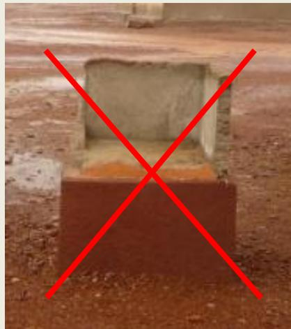
← Structure trop fragile, concentration en ciment insuffisante
