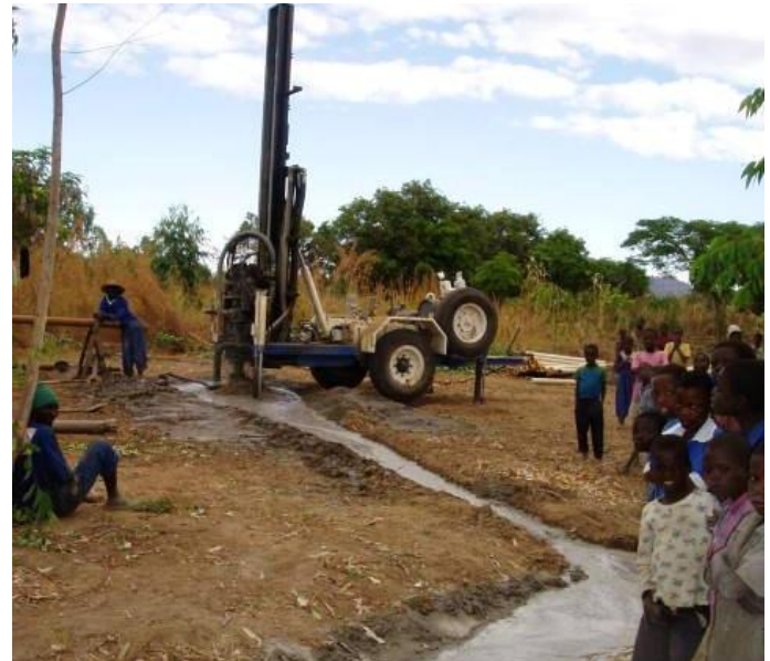
Figure 7: Controlling the discharging waters
