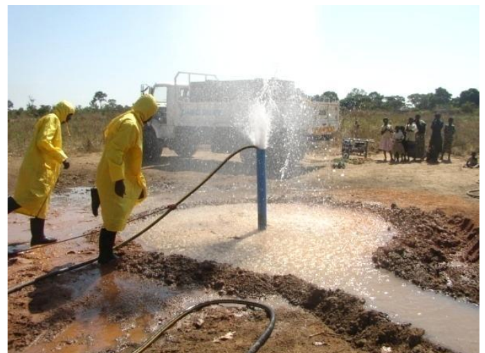
Figure 9: Cleaning the borehole with an air-jetting tool
