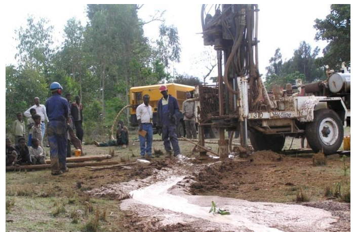
Figure 12: Drill rig with drilling fluid channel
