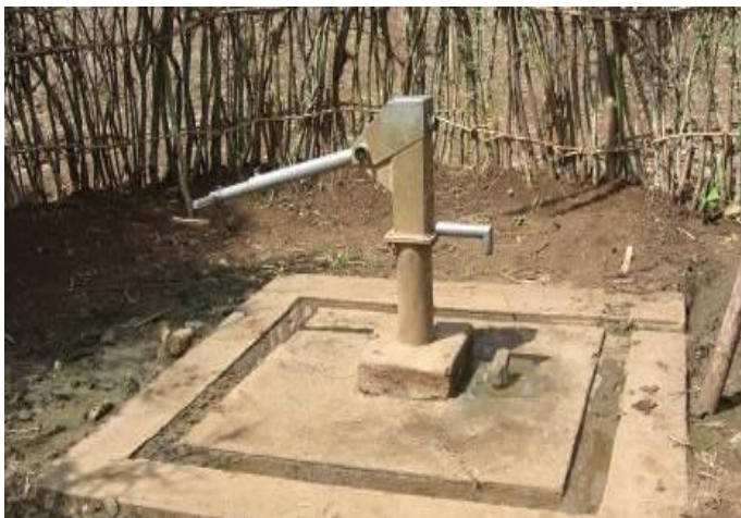
Figure 11: Rectangular pump platform (for wheelchair access)
