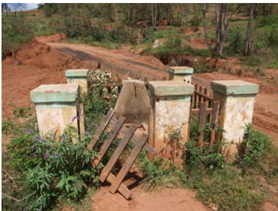
Standpipe abandoned due to lack of maintenance (Madagascar)
