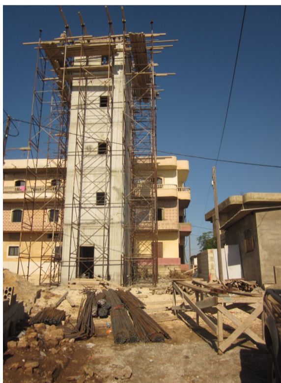
A water tower built by the NGO PUI_Akkar
