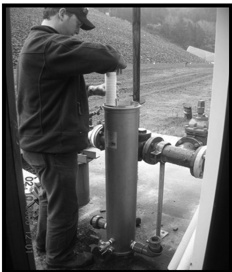
Figure 9a: Cartridge filter system
