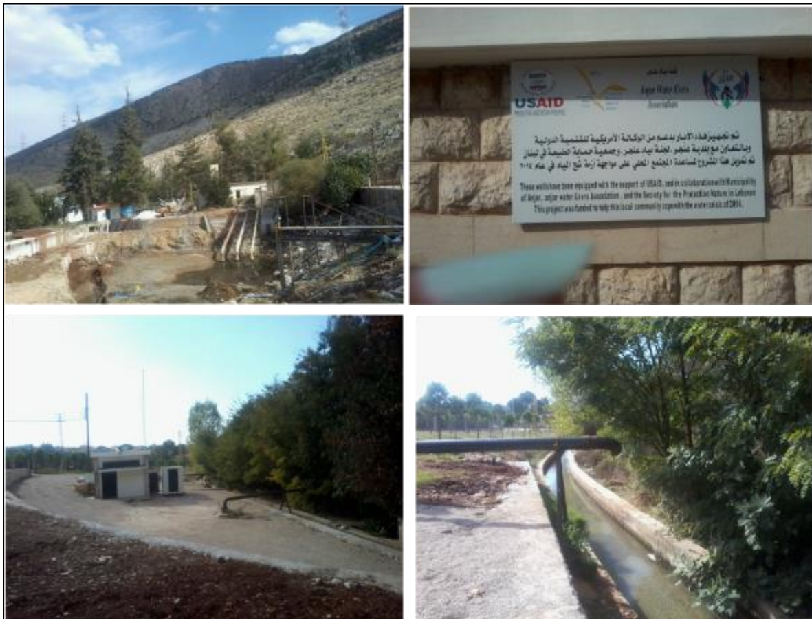
Figure 20: Anjar new collective irrigation wells.
