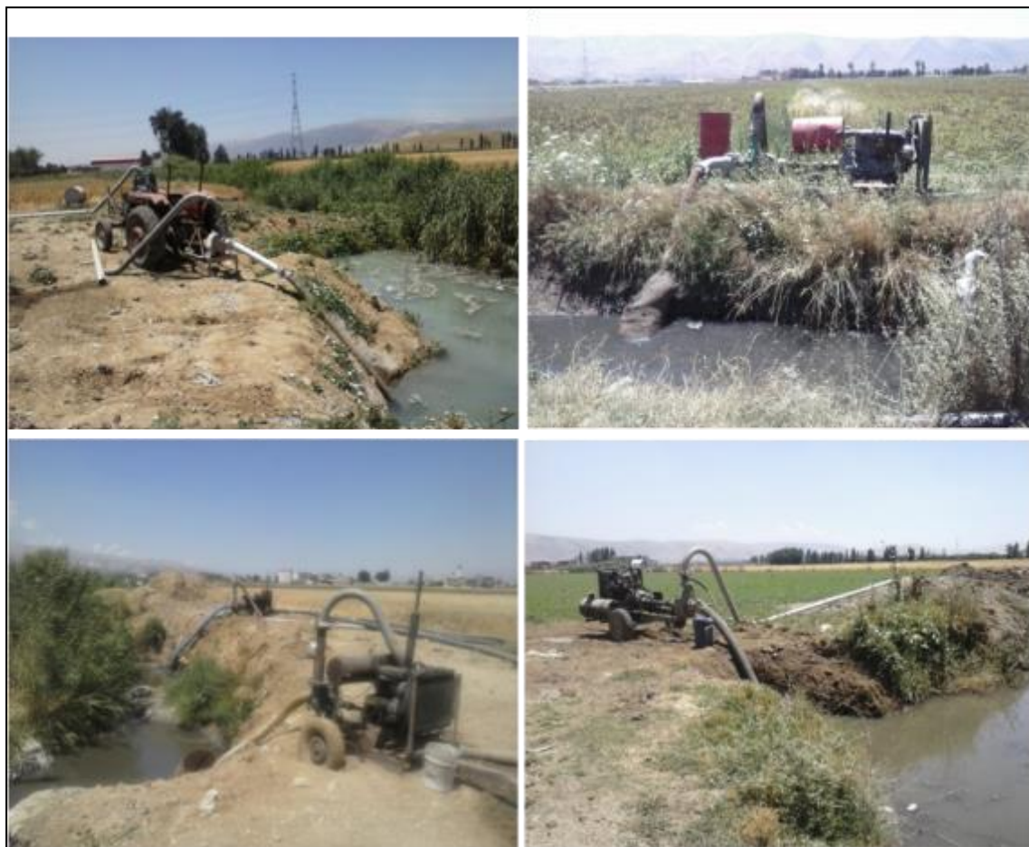
Note: Individual pumps abstracting polluted water from the Litani River at Barr Elias.
