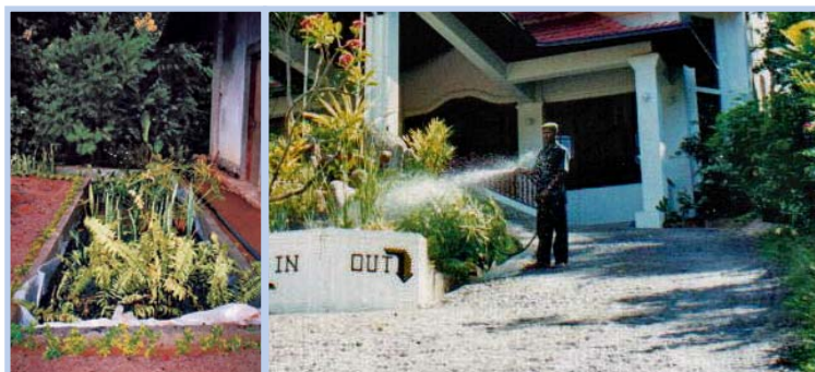
Photo 5-10: VFPF for greywater treatment at Swiss Residence Hotel in Kandy (left). The treated effluent is reused for gardening (right) (photo: Harindra Corea E.J.)
