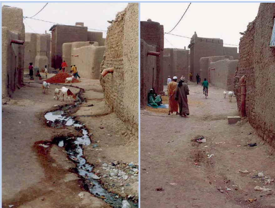
Photo 2-2: Djenné, Mali – The uncontrolled discharge of greywater has led to a deterioration of the streets, disease outbreaks, odour problems, and increased transport costs (left photo). The introduction of simple greywater infiltration systems as seen in the right photo on the wall, significantly improved the living conditions (photos: left, Alderlieste M.C., right, Langeveld J.G.)
