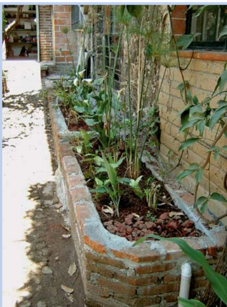
Photo 4-6: Horizontal-flow planted filter treating greywater of one household in Tepozlán, Mexico (photo: Sandec)
