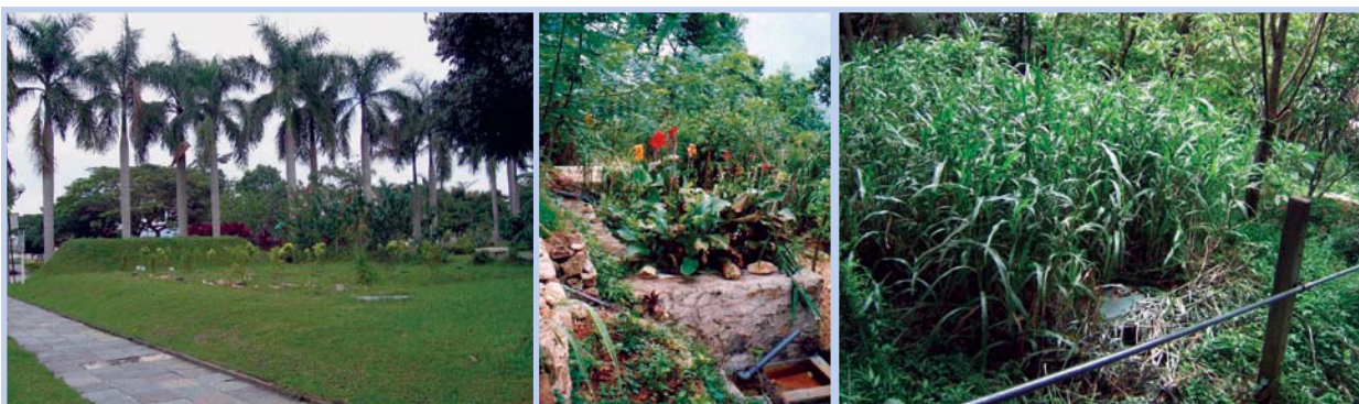
Photo 4-8: Left: Subsurface horizontal-flow filter (crushed limestone) fed by pretreated greywater from a neighbourhood of 45 persons in Kuching, Sarawak, Malaysia. The vegetation has an ornamental function only. The filter surface amounts to 2.8 m 2 per person equivalent (photo: Martin C.) Centre: HFPF with a simple swivelling elbow device (below, right) at the outlet for water level control in the filter, Sri Lanka (photo: Harindra Corea, E.J.) Right: HFPF (crushed rock) fed by pretreated greywater of four households (18 persons) in Monteverde, Costa Rica, with 1.7 m 2 /p specific surface. Coix lacryma-jobi , a locally available wetland plant, is used as emergent vegetation (photo: Sandec)
