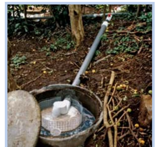
Photo 5-4: Settling tank (photo: Dallas S.)
