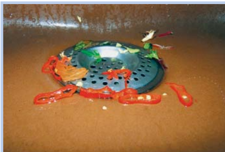
Photo 4-1: Kitchen sink screen to prevent solids from entering the treatment system (photo: Sandec)
