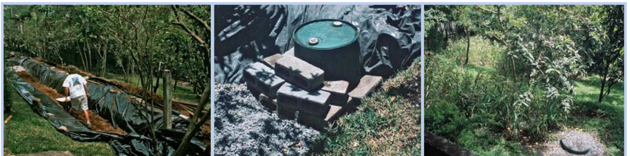
Photo 5-5: Build up of 1 st reedbed: Excavation (left), inlet drum (centre) and planted filter (right) (photos: Dallas S.)
