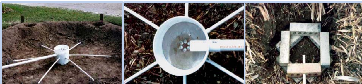
Photo 4-12: Greywater infiltration and irrigation system in Casa Juliana, Texas. Kitchen greywater is distributed via a hub to six small infiltration chambers irrigating papayas and bananas. The chambers are filled with mulch (photo: www.omick.net )
