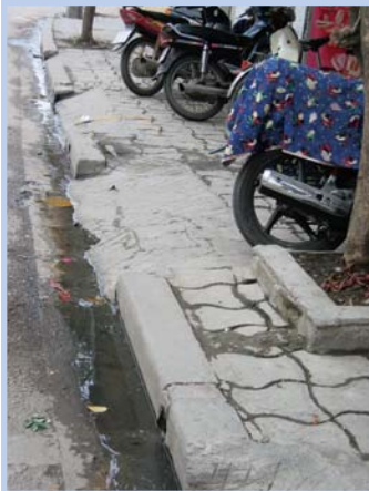
Photo 2-1: Greywater discharge in Hanoi (photo: Sandec)
