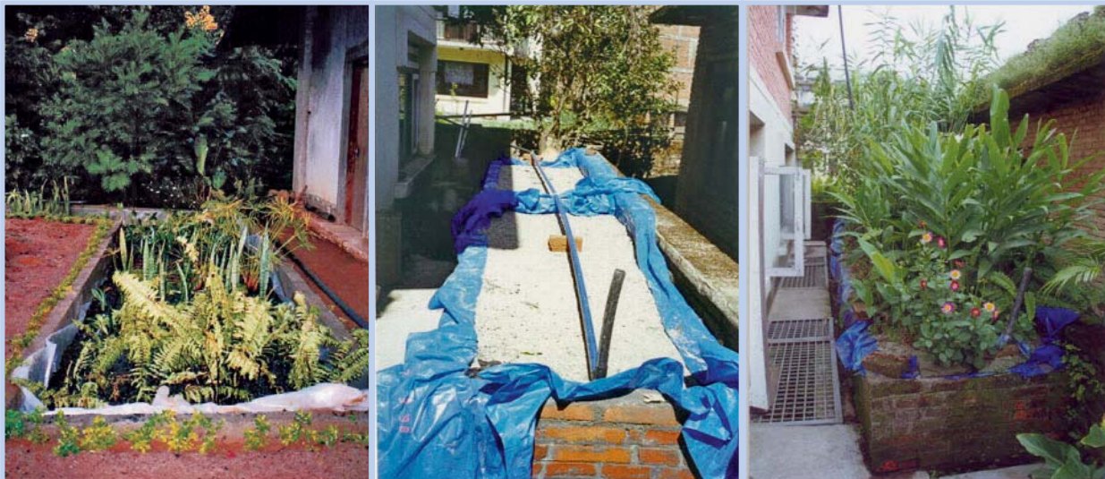
Photo 4-9: Left: VFPP treating kitchen and laundry greywater in a hotel in Sri Lanka, after pretreatment in a grease trap and septic tank (photo: Harindra Corea E.J.) Centre and right: VFPP implemented in a household in Kathmandu metropolis, Nepal, during construction and in operation. The constructed wetland has a surface of 6 m 2 and treats 500 l/d of mixed greywater after pretreatment in a sedimentation tank. The filter is planted with Phragmites karka and Canna spp. (photo: Shrestha R.R.)
