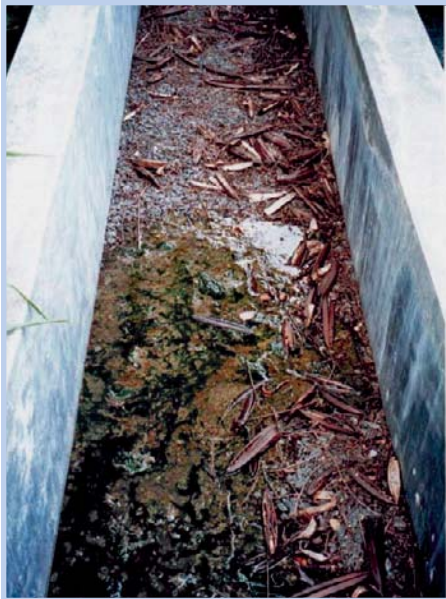
Photo 4-7: Clogging of the inlet zone of an unplanted horizontal-flow filter, indicating an overload of the inlet zone, possibly caused by the high L:W ratio, Sri Lanka (photo: Harindra Corea, E.J.)
