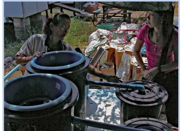
Photo 4-2: Mosquito nets used as coarse filter in a combined sedimentation/filtration system for greywater treatment in Bangkok's channel communities. The light blue basin can be removed and easily cleaned (photo: Sandec)
