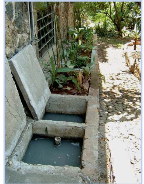
Photo 4-3: Grease trap ahead of horizontal-flow planted filter installed in Tepoztlán, Mexico (photo: Sandec)
