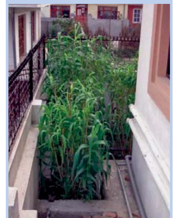
Photo 5-6: Vertical-flow planted filter shortly after completion (above) and in use (below) (photos: Shrestha R.R.)
