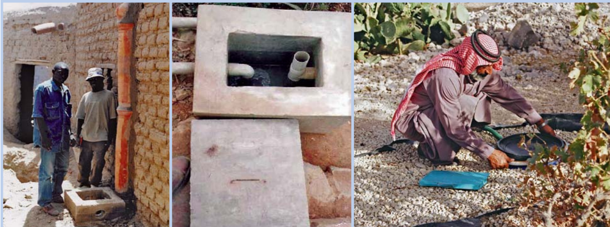
Photo 4-4: Left: Grease and grit trap used as primary treatment unit in a greywater infiltration system in Djenné, Mali. Given its small size, the trap often clogs, thus jeopardising the subsequent infiltration system (photo: Alderlieste M.) Centre: Grease trap implemented in a household greywater irrigation system in Peru. The trap is undersized, vertical baffles are missing, resulting in clogging of the subsequent planted filter (photo: Garcia O.) Right: Buried, recycled 160-litre plastic barrel used as grease trap and grit chamber ahead of an unplanted horizontal-flow gravel filter in Jordan (photo: Kassay J., IDRC)
