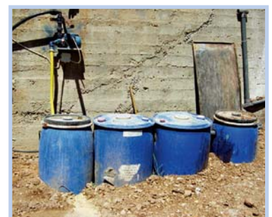
Photo 4-5: Four-barrel up-flow anaerobic filter implemented in Jordan. Two tanks of 220-litre capacity each filled with gravel media acting as anaerobic filters are inserted between a sedimentation and a final storage tank (photo: Redwood M., IDRC)
