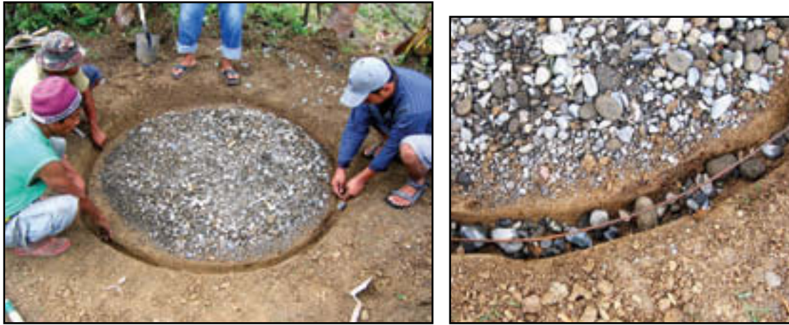
Fig. 49-50: Excavating the base and Adding gravel
