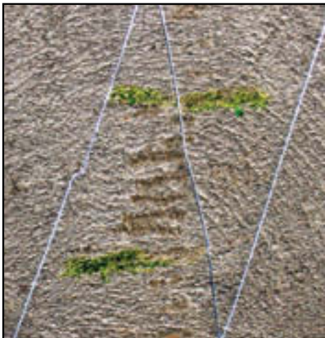
Fig. 65: Marking horizontal wire placement
