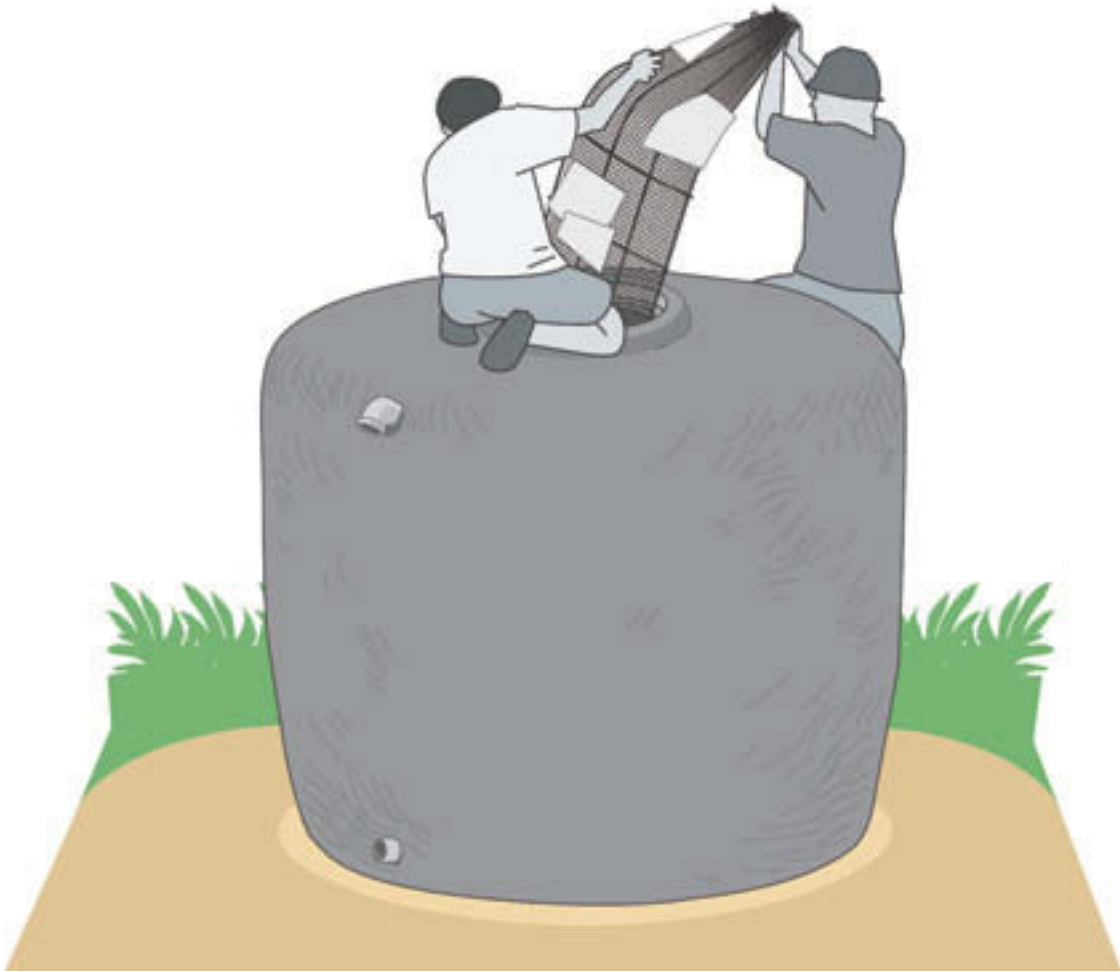
Fig. 42: Removing the form
