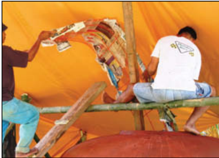
Fig. 70: Removing the form
