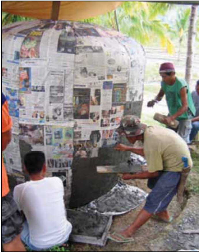
Fig. 57: Plastering the first layer
