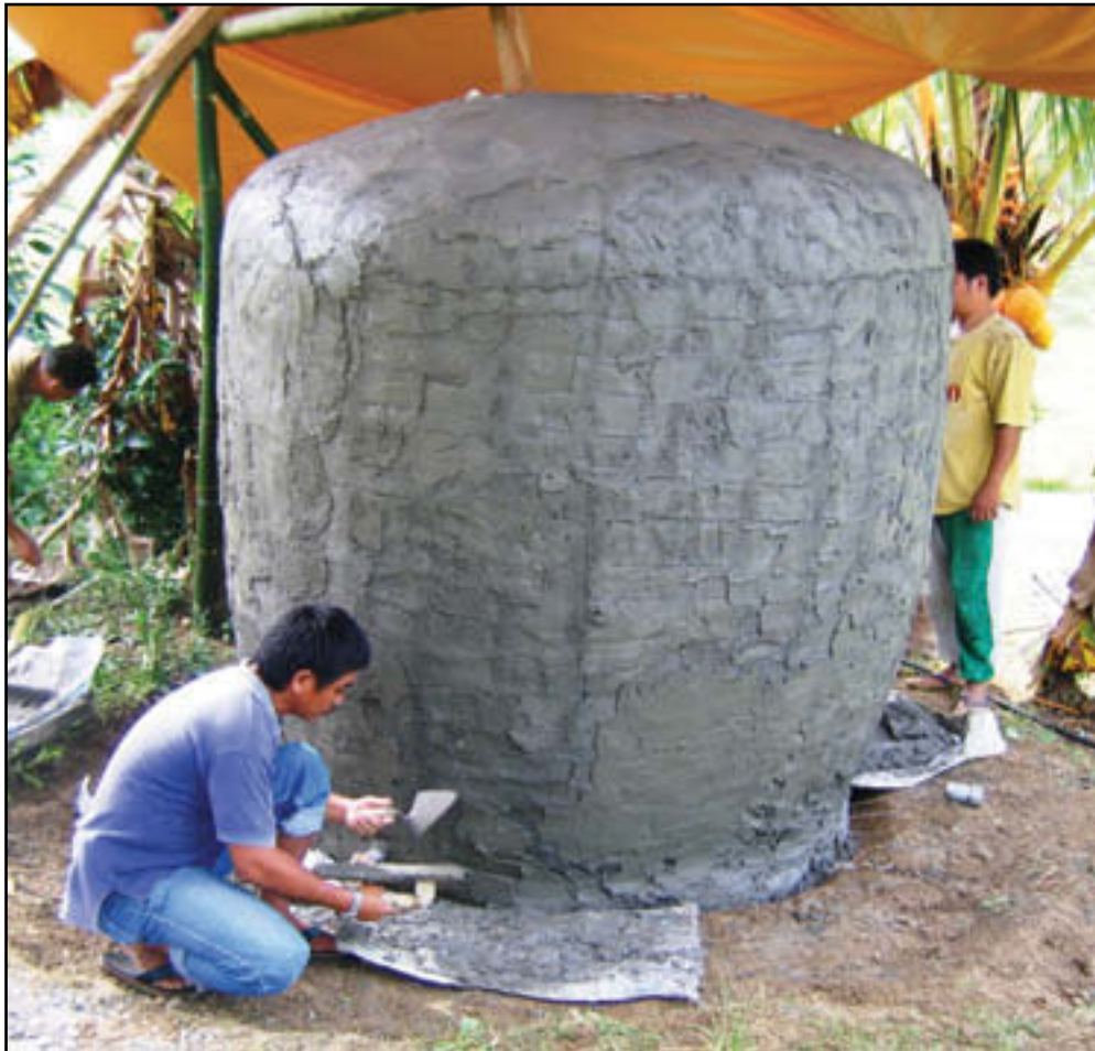
Fig. 60: Plastering the second layer
