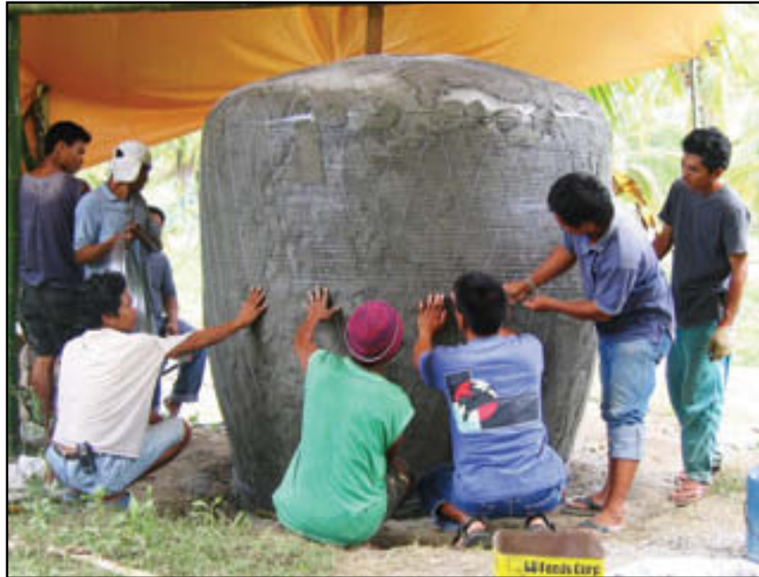
Fig. 66: Horizontal wire reinforcement
