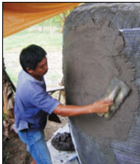
Fig. 67: Applying the final layer
