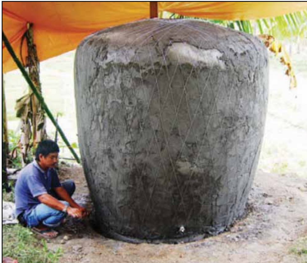
Fig. 63: Completed vertical wire reinforcement
