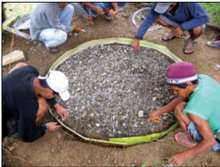
Fig. 51: Adding base reinforcement
