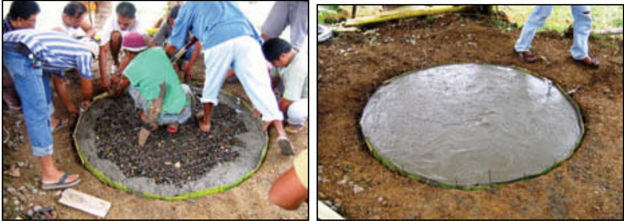
Figs. 52-53: Pouring cement and The completed base
