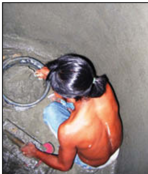
Fig. 71: Plastering the inside of the tank
