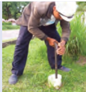
Valve turning for control of distribution
