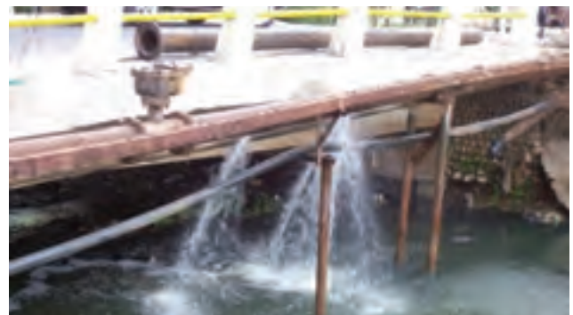
More obvious leaks
