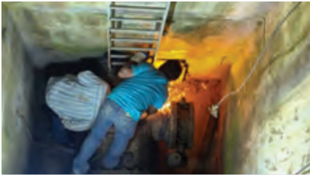
Installing a 600 mm butterfly valve
