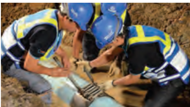
Repairing a distribution leak (e)
