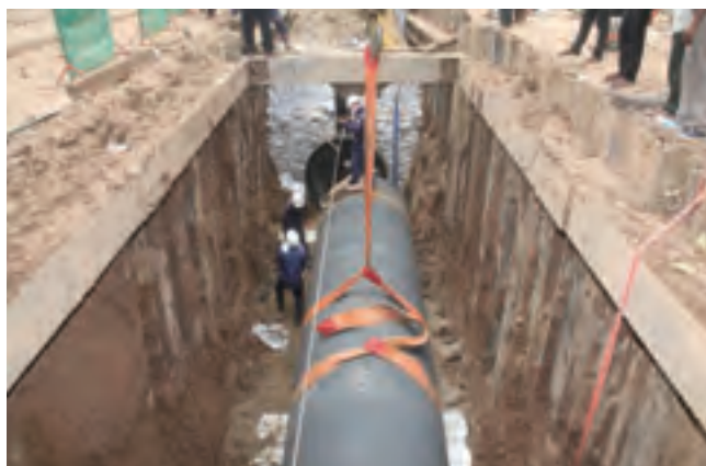
Daytime construction of transmission mains
