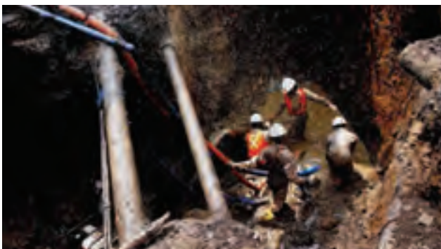
Repairing a distribution leak (c): not easy at great depth
