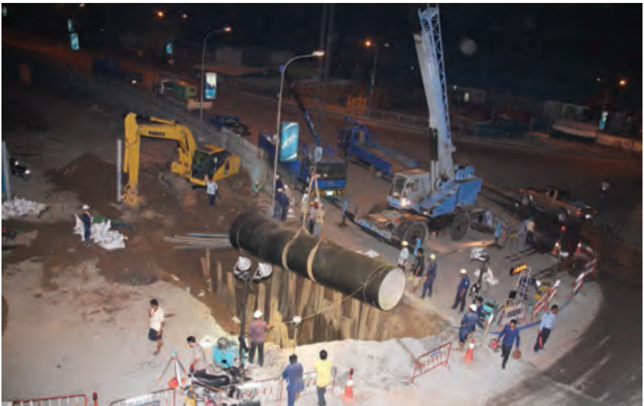
Night-time construction of transmission mains
