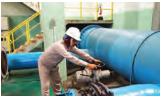
Valve turning under intermittent supply
