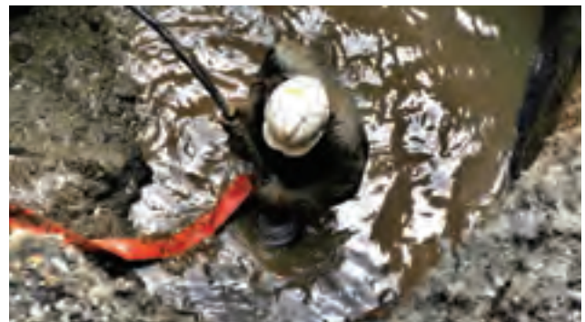
Repairing a distribution leak (b)
