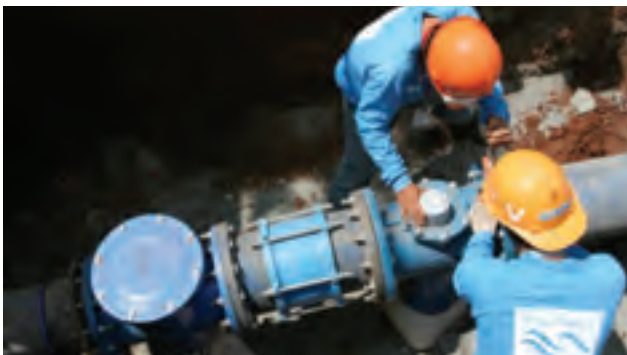
Repairing a distribution leak (a)
